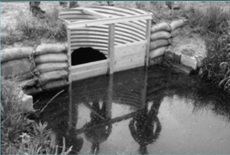
**Fig. 2** *Controlled drainage system showing flashboard riser*
